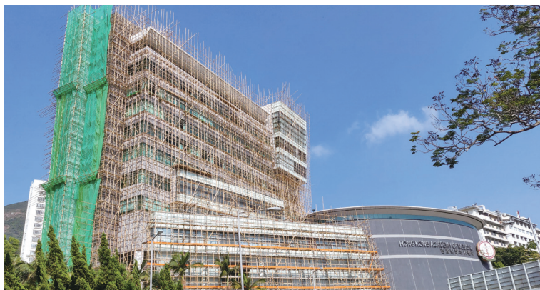
The second phase of works include repairing of the external wall of the main building and canopy at the main entrance. 第二期工程包括修葺主大樓的外牆及大樓正門上蓋。
